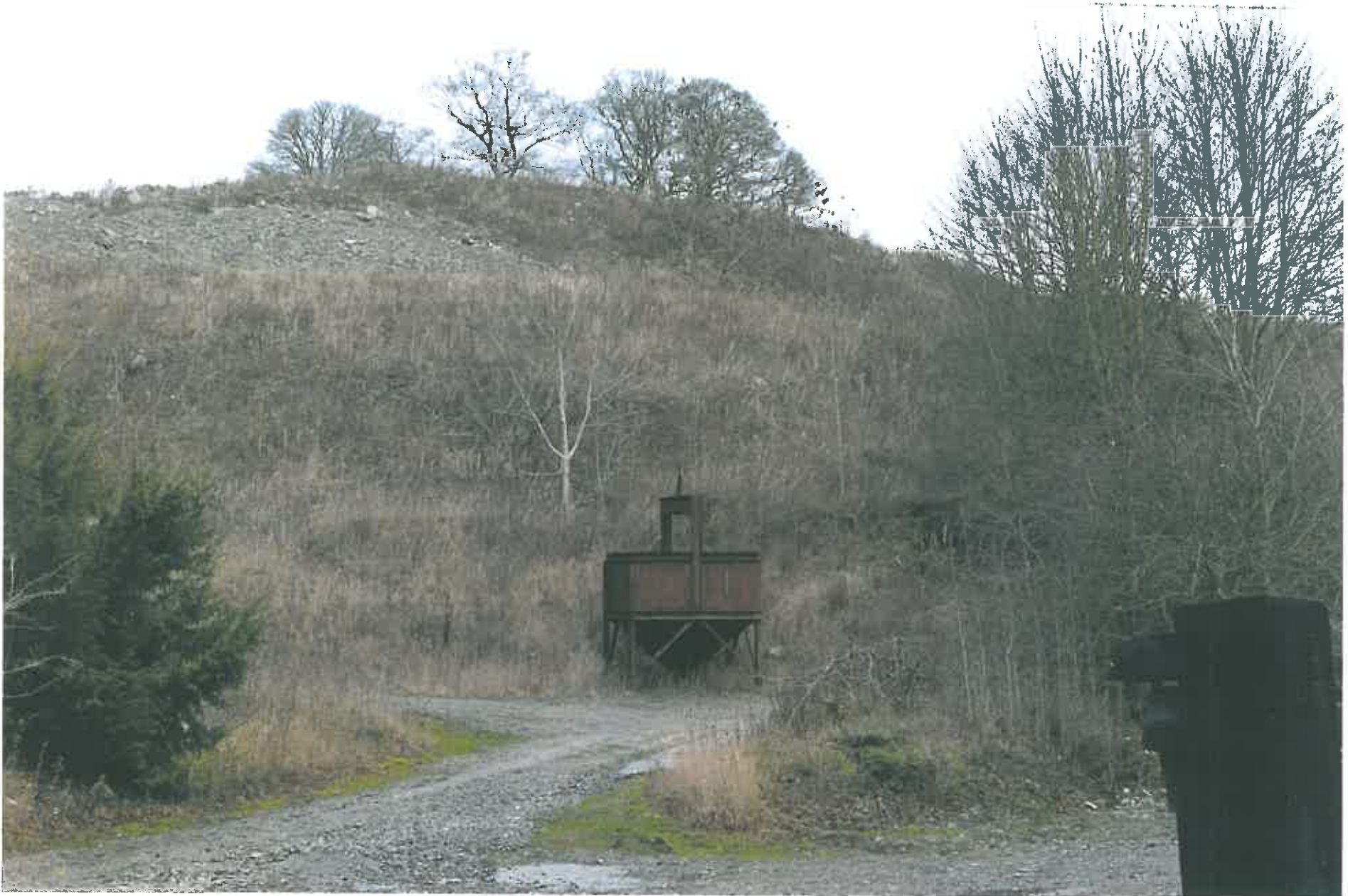
Backdale Quarry viewpoint E(2): Looking north east towards the eastern overburden mound form diverted public footpath
